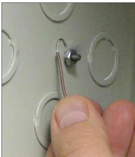
Fig. 5: Connect ground wire to grounding screw.
